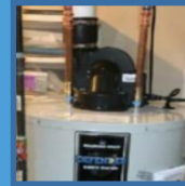
Gas Evacuation Systems
