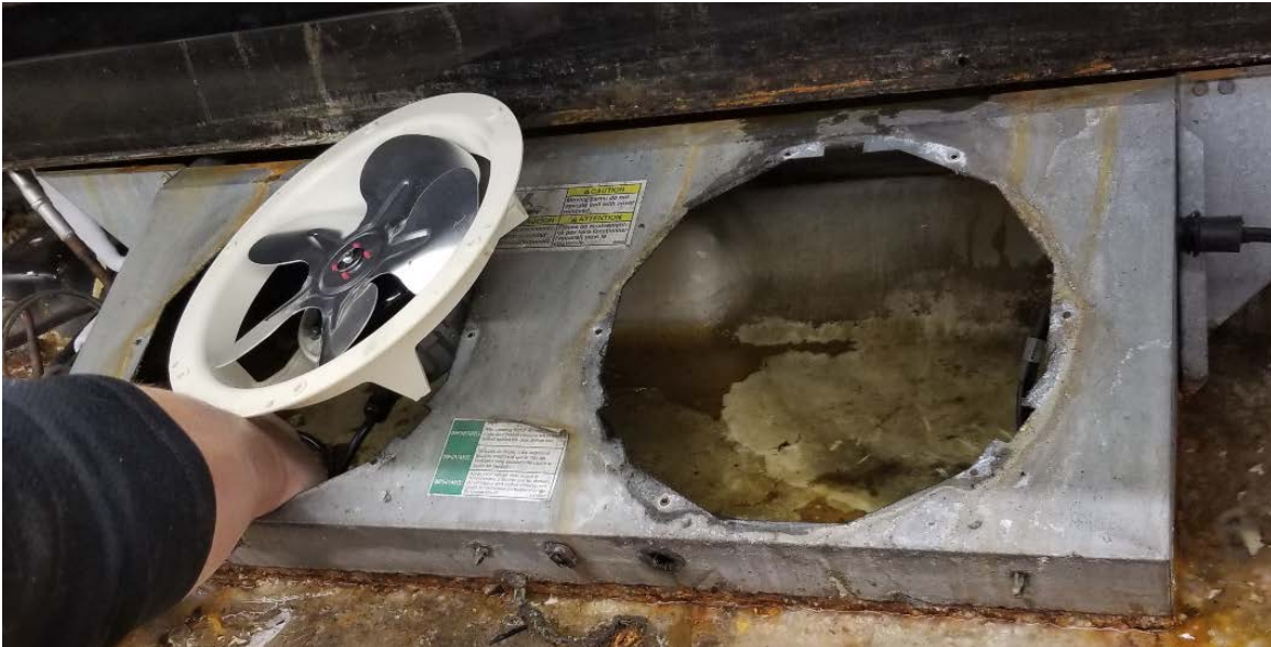
FIGURE 3. INSTALLATION OF A RETROFIT PMSM FAN
